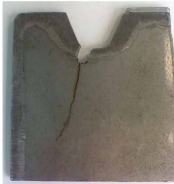
Figure 7—Cross Section of an RTJ Flange with Cracking from the Inner Corner that Extended Deeply into the Cr-Mo Base Metal
